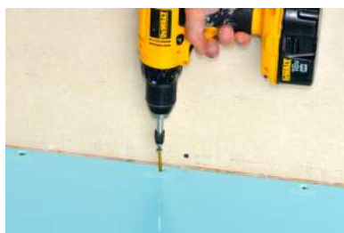
Drive perimeter screws so they are snug, but not so tight as to unlevel the base.
