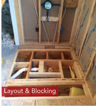
Install Base & Drain
