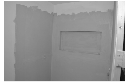
Niche joints and corners require embedded tape protection, plus two full coats of waterproofing.
