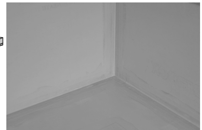
Allow the first full "tanking" coat to dry before topping it with a second full coat.
