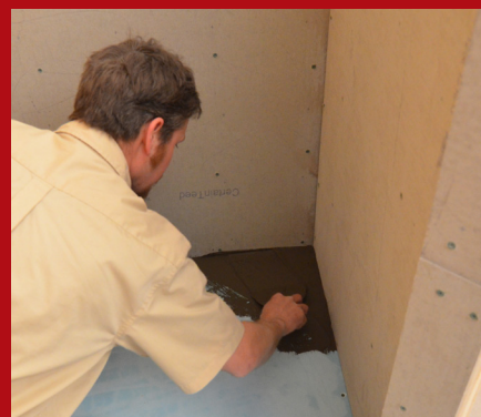
Spread thinset with a trowel, making sure it is high in the corner to yield a 1/4" per foot slope.
