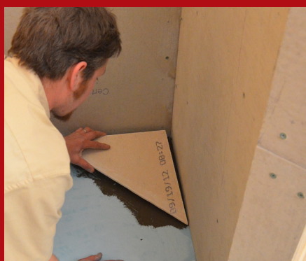
Apply thinset to the underside of the extension panel, then gently press it into position.
