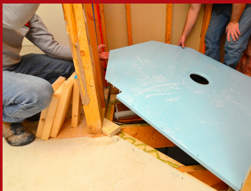
After making sure the base rests level and even on all blocking and joists, install it with adhesive and screws.
