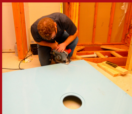
Cut the corners of your TrueDEK Classic shower base using a circular saw and carbide blade.
