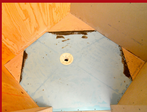
Thinset is a good gap filler and can be used to smooth transitions from extension panels to the shower base.
