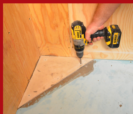
Allow thinset to dry a while, then, once it's firm, drill countersunk pilot holes and drive screws.
