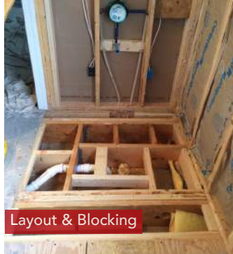
Install Base & Drain
