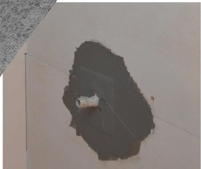
**Embed a supply gasket around supply pipes in the wet area for shower heads, hand held devices, and jets or sprays.**
